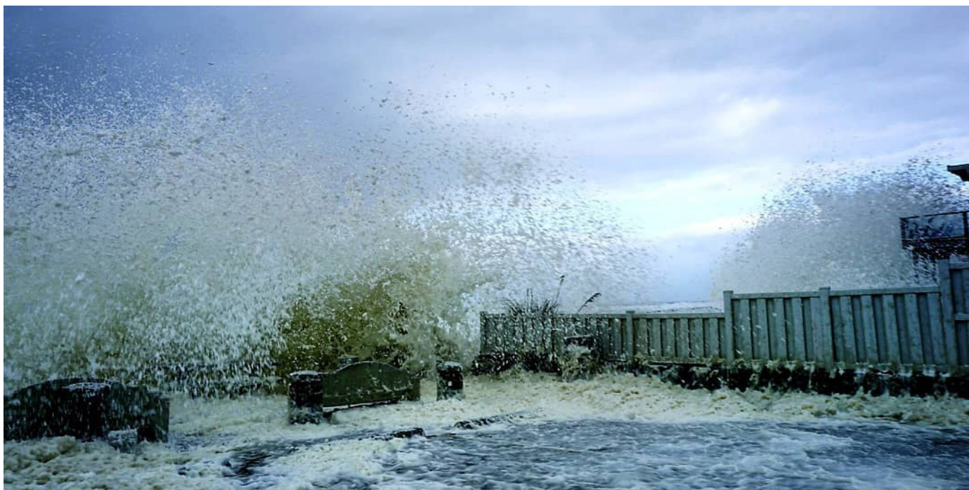
Waves crash over seawall during winter storm, inundating public space and coastal homes.
